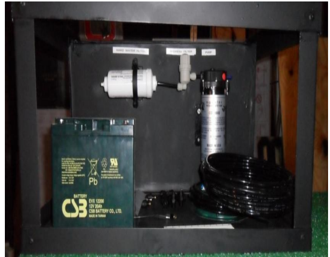
Figure 3. Waterproof Housing of Filters, Pump, and Battery
